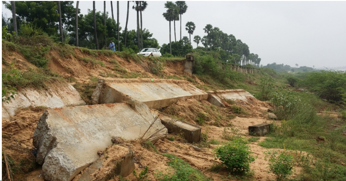
Damaged Retaining wall
